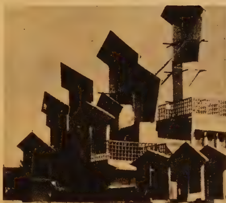
Rooftop wind scoops, Hyderabad, Sind. A rare climatic paradox—high humidities superimposed on Arabian Desert temperatures—makes ventilation mandatory. These wind scoops are oriented to prevailing breezes.
